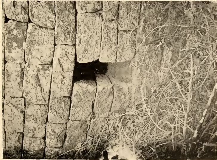
EXTERIOR OF A DRAIN, ELLIPTICAL TEMPLE
