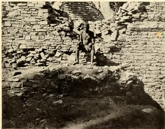
JOINT BETWEEN ORIGINAL AND RECONSTRUCTED WALLS, Nos. 11 & 12 ENCLOSURE, ELLIPTICAL TEMPLE
